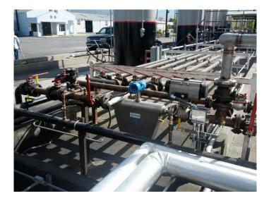
by using the batch controller, control valve and Coriolis meter for the batching process, the customer can now dial in the desired amount of individual components and then walk away. These flow meters were also integrated into a local display, a Precision Digital Consolidator which displays values of tank levels and flow rate.
