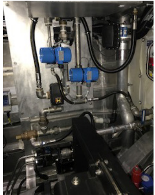
The very small footprint of the AW-Lake Turbine Flow Meters met the installation challenge posed by the limited space of the bottom deck of the fire boats.
