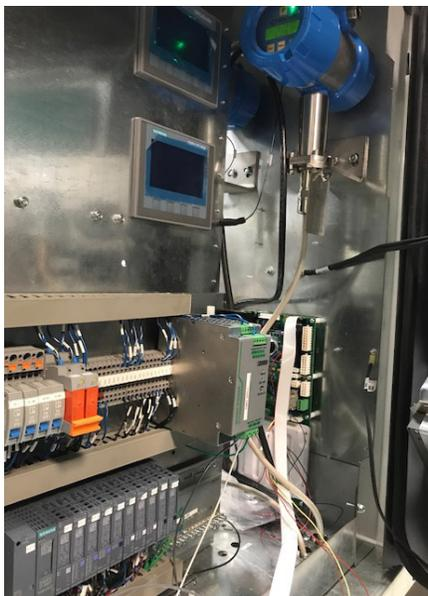
Rear view of control system with IO cards and dispensing controls
