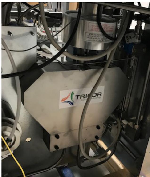
Rear view of hydrogen pumping station showing TCM-0450 High Pressure MID-002 / OIML certified Coriolis meter.
