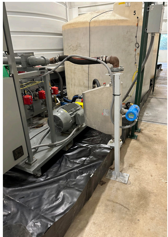
TCM-65K Coriolis meter measuring raw product arriving via tanker trucks and finished product loading onto tanker trucks for delivery to distribution sites.
